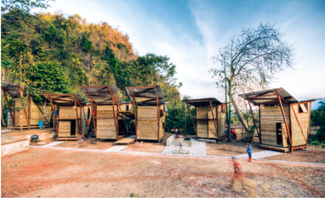
Safe Haven - orphanage, Tyin Tegnestue Architects Ban Tha Song Yang, Noh Bo, Thailand, 2009 Client: Safe Haven Orphanage with the assistance of Trondheim University (NTNU), Professors Sami Rintala and Hans Skorte; Ole Jørgen Edna © Pasi Aalto
